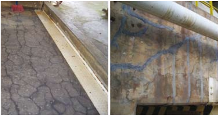
Figure 3: Cracks due to excessive vibration of equipment.
