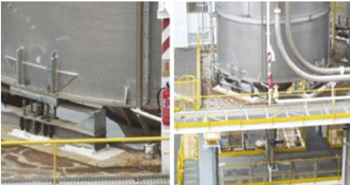
Figure 2: Cracks on structures supporting equipment.
